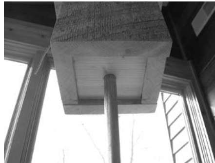
Bottom mount conduit method used by Roy.
