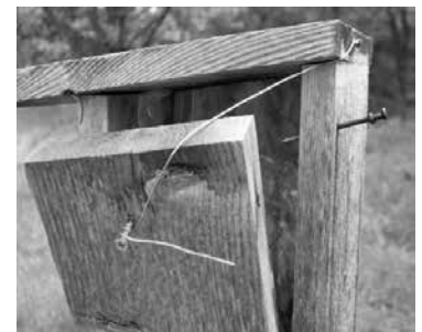
Fig. 5. Wiring boxes open to prevent woodpecker damage.
