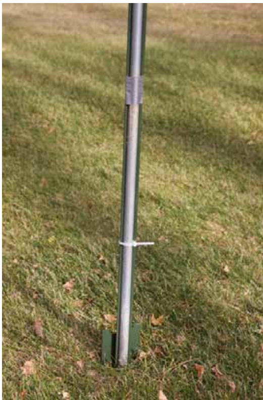
2. A 4-ft. green steel post will provide support for a 6-ft. pole. Tape keeps pole from turning.
