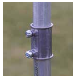
5. A set-screw coupling is used to join to conduit pipe sections of equal diameter.
