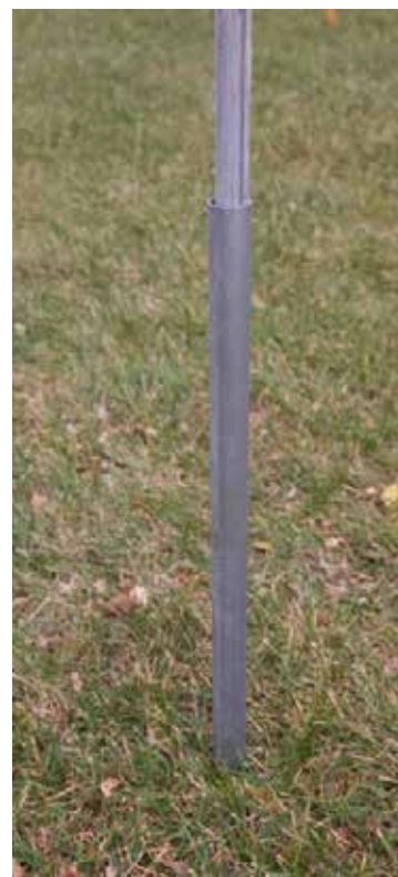
3. A smaller diameter pole can be inserted into a 2.5-ft. anchor pipe.
